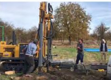
深水井施工 Deep well construction
