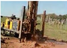
深水井施工 Deep well construction
