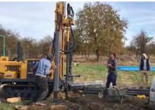
深水井施工 Deep well construction
