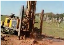
深水井施工 Deep well construction
