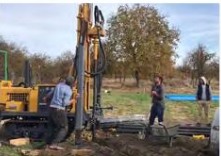
深水井施工 Deep well construction
