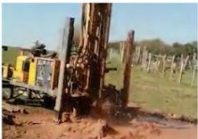
深水井施工 Deep well construction
